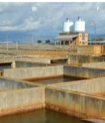
A : SOCIAL DEVELOPMENT OF CHILDREN B : WATER SUPPLY PIPES C : AJAX VS SANTOS AT ATHLONE STADIUM D : BUILDING GREEN POINT STADIUM E : KOEBERG INTERCHANGE F : FAURE WATER TREATMENT WORKS
